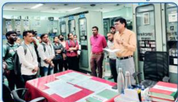
Mahatransco Mahape - 220 KV 22 KV Substation
